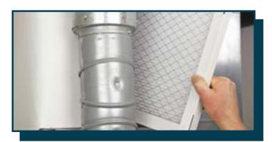
In addition to changing the air filter, it's important to schedule a routine inspection of your home's HVAC system. This includes an inspection of the appliances themselves and any connecting ducts. Dust, dander, and mold can accumulate in the ducts and spread throughout the home, which can lead to health issues, including respiratory problems.
